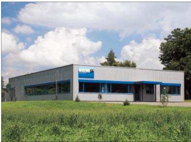
The new ultra-modern Wibemo plant, located right in the open countryside.
